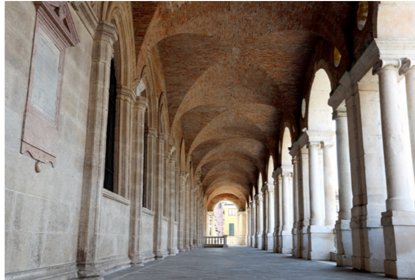
▲ Gothic arches or a loggia.
